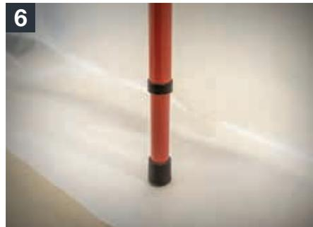
**6** Place sheeting under the reinforced, tensioned foot to hold sheeting in place.
