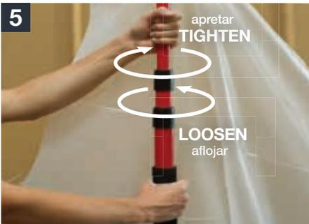
**5** Twist pole sections counter-clockwise to loosen. Adjust height, then twist pole sections clockwise to tighten. The tensioned foot will keep continual pressure on the floor and ceiling, locking the pole & sheeting in place.
